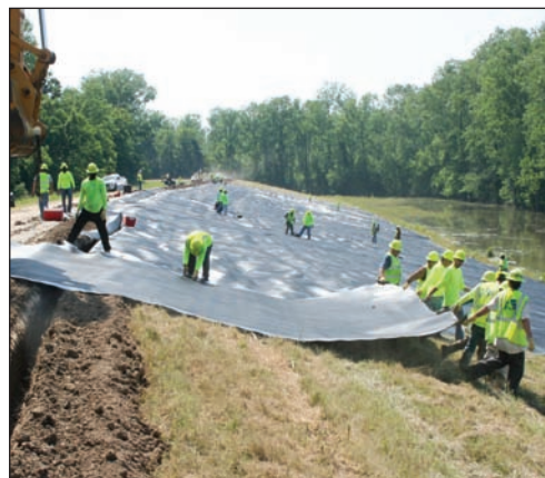
Poly sheeting being installed on landside slope of YBW Levee.
