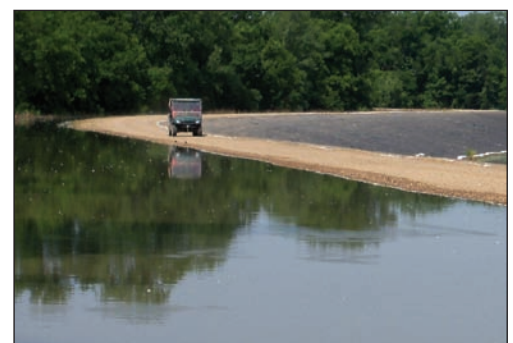
Water within 4" of the top of the YBW Levee.
