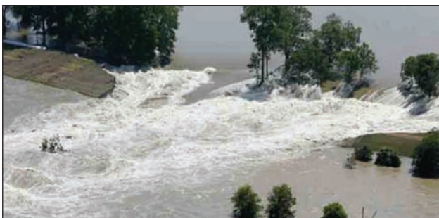
Non-MR&T Levee overtopping and failing during 2011 flood.
