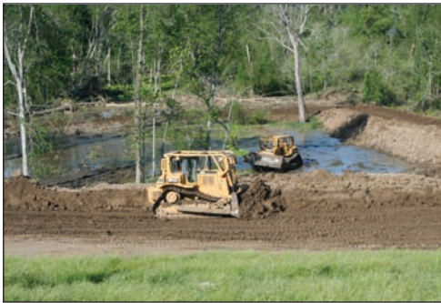
Corps building earthen water berm around sandboils at Buck Chute.
