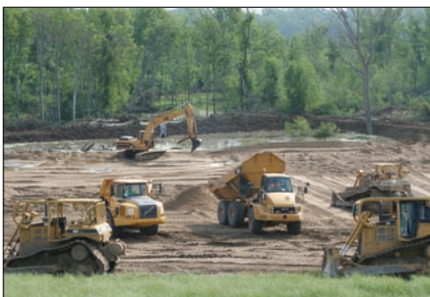
Corps filling Buck Chute sandboil area with sand.
